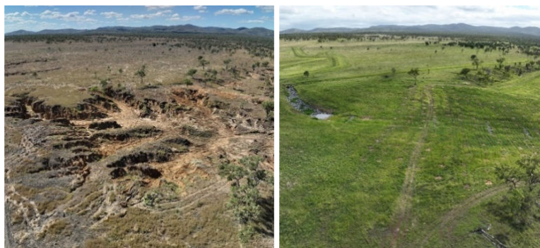
Figure 2. Example of LRP alluvial gully site before (May 2023) and after (March 2024) remediation. Actions included reshaping, diversion bank and associated rock chutes, porous rock check dams, soil amelioration, revegetation, fencing, and grazing management.
