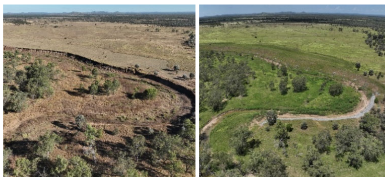
Figure 3. Example of LRP streambank site before (Nov 2024) and after (March 2025) rehabilitation. Actions included vertical bank battering and construction of rock chute, batter drains, bunds, rock beaching, and pile fields; soil amelioration, revegetation, fencing, and grazing management.
